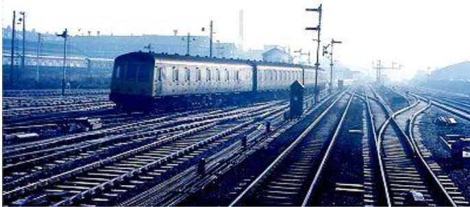
A Class 116 returning to Cricklewood depot after a morning rush hour run From Luton to Moorgate. Taken from the picture from the cab of a class 25 on the goods line. About 9.00am, January 1975. Photos: Arno Brooks
